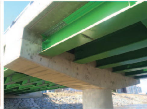
Integrated Bridge with Buried Girder Type
